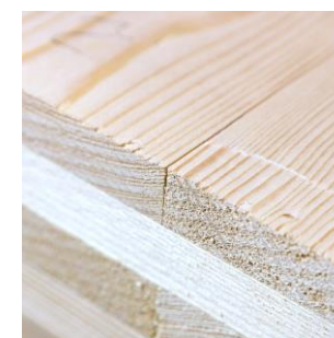
Crack on the plate
